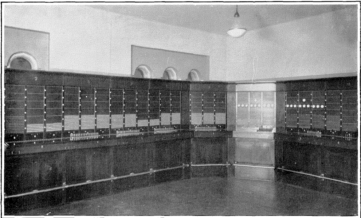
Figure 6—Operating Room—Subscriber boards on the left side, toll boards on the right side.
