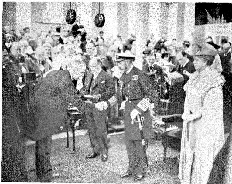
Figure 3—H.M. King George V Laying the Foundation Stone for Lloyds New Building, London.
